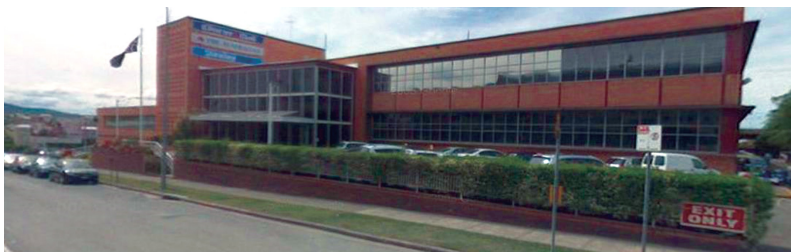
QNPL's offices at 41 Campbell Street Bowen Hills in Queensland - News Limited's 1° energy saving program is being implemented using Ilum-a-Lite technology and ecoBright® service with impressive results. Photo is © 2010 Google and reproduced with kind permission.
