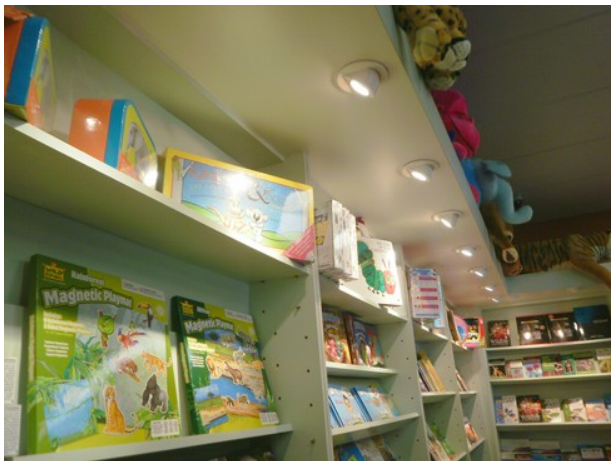
Part of the product display setup in the Zoo's Retail stores - the ecoBright® R4 LED solution is seen easily retrofitted into existing Halogen fittings.
