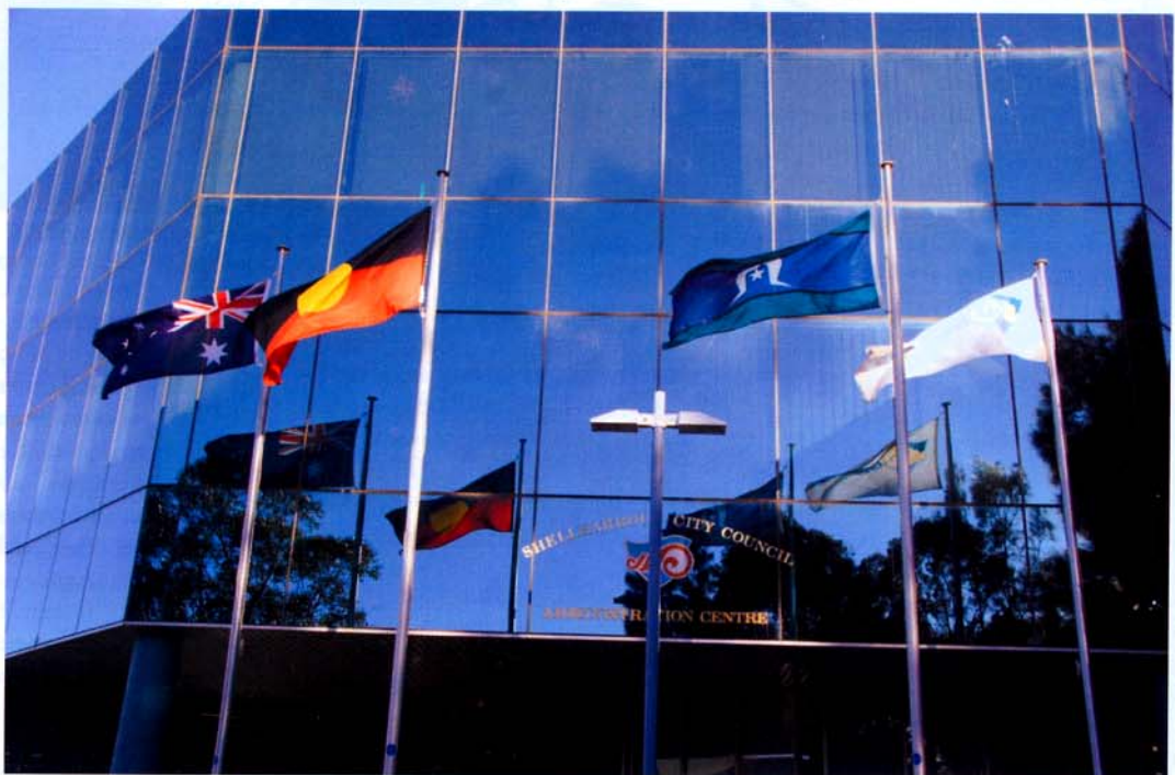
Lamerton House in Shellharbour . . . 30 per cent energy saving by installing T5
