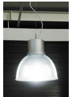
A close-up of the ecobulb® 65W Self Ballasted CFL lamp and customised pendant fitting.
