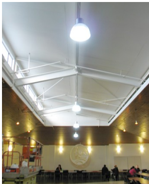
The Cafeteria at Te Wānanga fitted with the new ecobulb® 65W Self Ballasted CFL lamps in pendant fittings.
