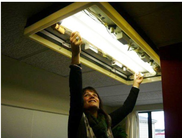
Nastasha of SBN showing how simple it is to fit the ecoBright® T5 adaptor, replacing 52W T12 lamp and ballast with 31W T5 lamp and ecoBright® T5 adaptor as ballast. That's a saving of over 40% per lamp!!
